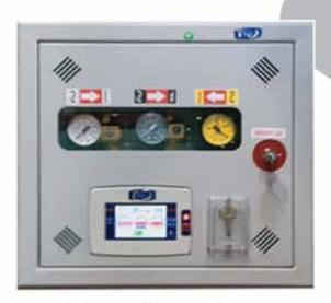
interventions. There should be an emergency intervention system on the panel. In this way, in case of emergency; cover can be opened and breakable glass should allow for rapid intervention.
